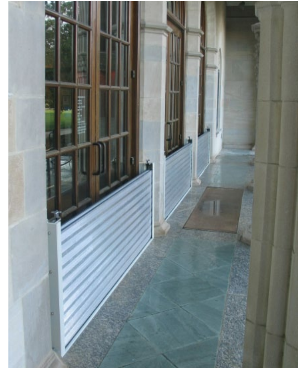
3. Flood shields deployed (close-up)
